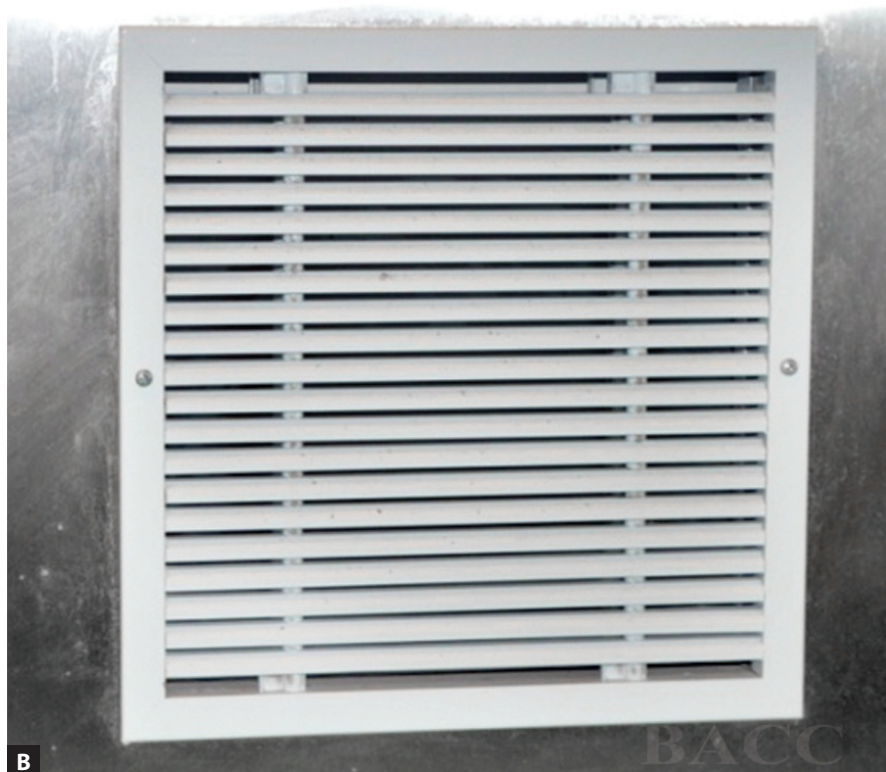
Figs. 2A and B: Air handling unit.
